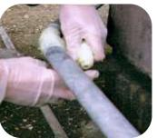
A chemical process line had started to leak due to a hole forming in the pipe wall, the surface was mechanically abraded and 108 Pipe Repair Tape wrapped around the pipe work to a minimum thickness of 12mm over the repair area.
