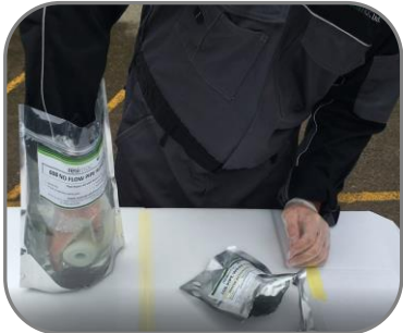
Using the kit bag supplied, drop the roll into cold water for a maximum 30 seconds and squeeze several times
