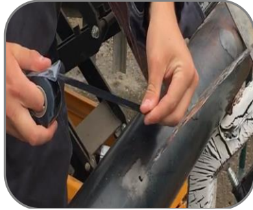
Silicon amalgamating tape used to stop the pressure around the repair
