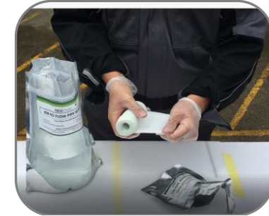
Once the leak has been stopped, take the 108 pipe repair tape out of the sachet
