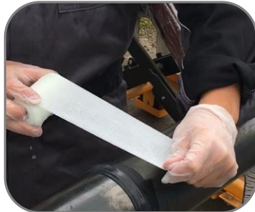
Position the tape over the repair surface, off centre
