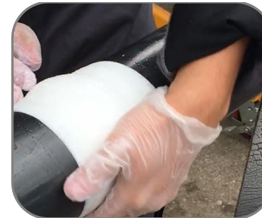
Wrap the bandage over the leak as many times as possible, building the thickness of the bandage over the hole or crack
