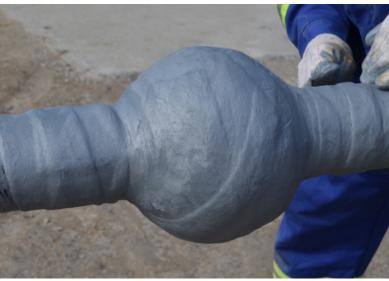
Use of Fill-Pro<sup>™</sup> PM-GP profiling mastic creates a uniform profile for the application of Trenton Wax-Tape<sup>®</sup> anticorrosion wrap.
