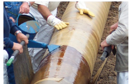
A thin coating of Innercoat can then be applied over the Guard-Wrap for additional protection.
