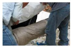
A second continuous wrap of Seal-Wrap applied directly over the first wrap.
