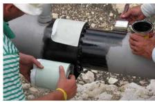
First layer of Double-Faced Adhesive is applied to the casing, Seal-Wrap Primer being applied to the carrier.
