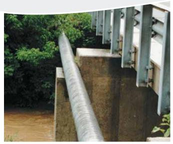
Wax-Tape<sup>®</sup> #2 anticorrosion wrap has a proven history over three decades of successful field applications. It is used with Trenton primers, profiling mastics and outerwraps to create the Trenton Wax-Tape<sup>®</sup> System.
