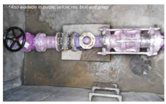
Wax-Tape<sup>®</sup> #2 anticorrosion wrap is available in many colors. This pipe is wrapped in purple tape, often used in the water industry. Wax-Tape #2 wrap meets AWWA C217 2016 standards.
