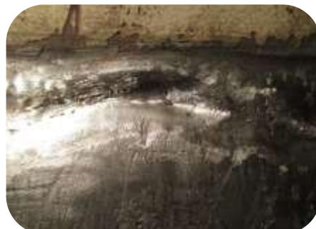
Sea water pipe spool reducer was internally corroded and in need of repair, surfaces were mechanically abraded and rebuilt using 201 Ceramic Repair Paste
