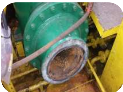
Sea water pipe spool reducer was internally corroded and in need of repair, surfaces were mechanically abraded and rebuilt using 201 Ceramic Repair Paste
