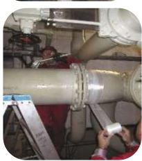
301 Epoxy Resin Hardener was brush applied to pipework situated in a plant room. The pipe wall thickness had deteriorated over time and the pipes were weeping hot water onto the floor below, Due to the fragile state of the pipes surface preparation was carried out using hand held wire brushes. Once the surface of the pipe had dried 301 Epoxy Resin and Hardener was applied at 1mm wet film thickness to the pipe surface and wrapped 3 times using 100mm glass tape
