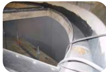
Chemical powder process vessel and chute were lined with 3mm of 209 EIP PU.
