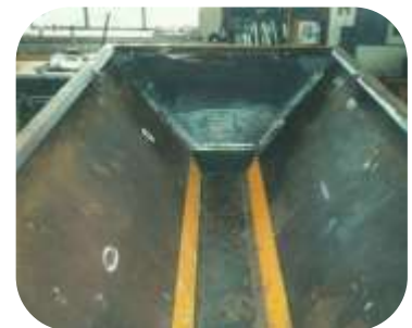
Aggregate sieve abrasive blast cleaned and relined with 3 coats of 209 EIP PU
